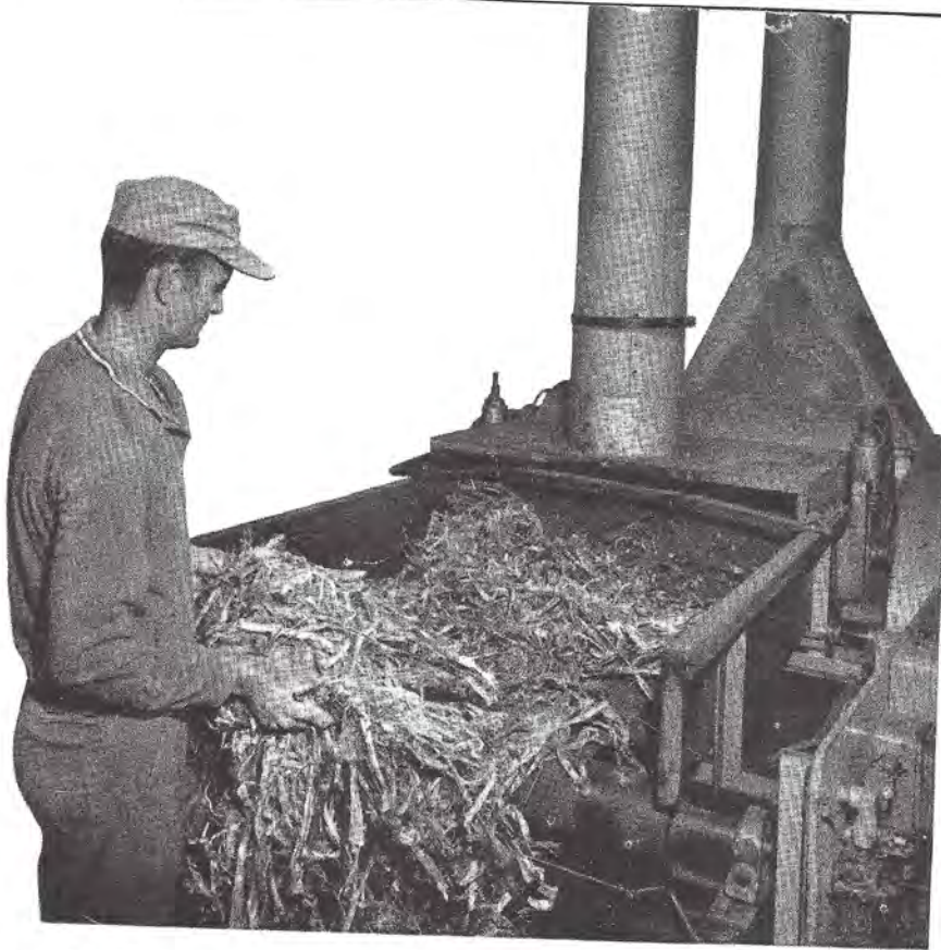
Above, jute is fed onto belt which carries it into picker. Inside, the jute is cleaned of dust, dirt and other debris. Below, jute cords come from a cording machine. Observing are Charles J. Wolford, left, Esso representative, and Jay E. Tollstrup, right, Nupak production manager.
